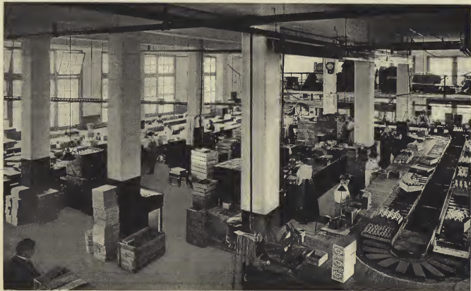
General View of Adhesive Department, Bottling Floor.
